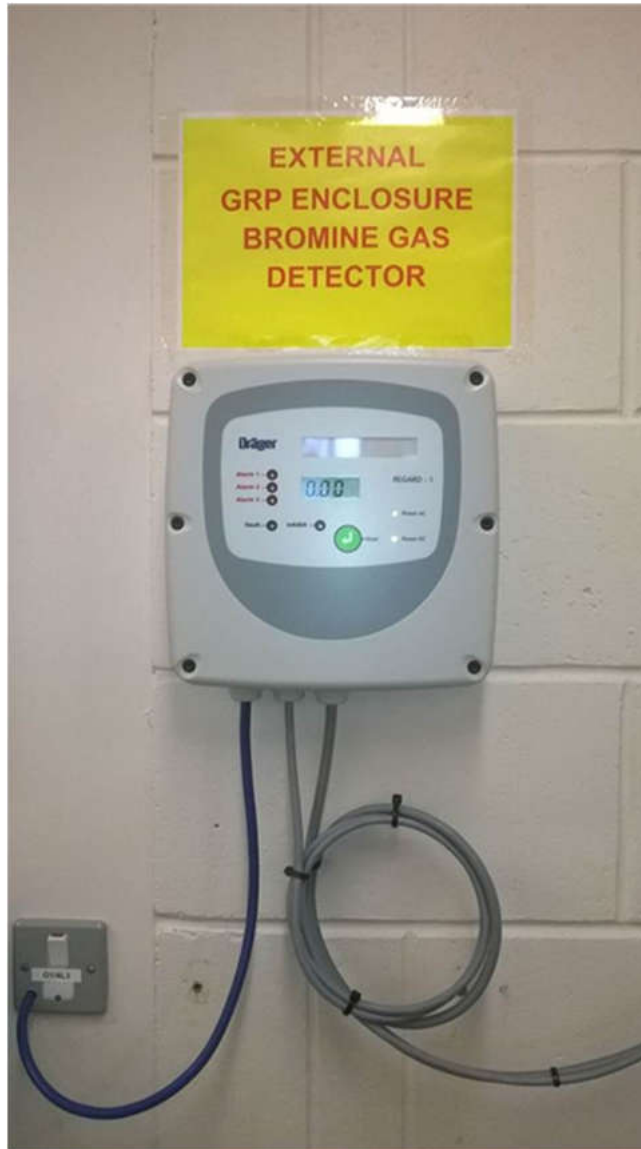
The Bromine gas detector display inside the PNDC building
